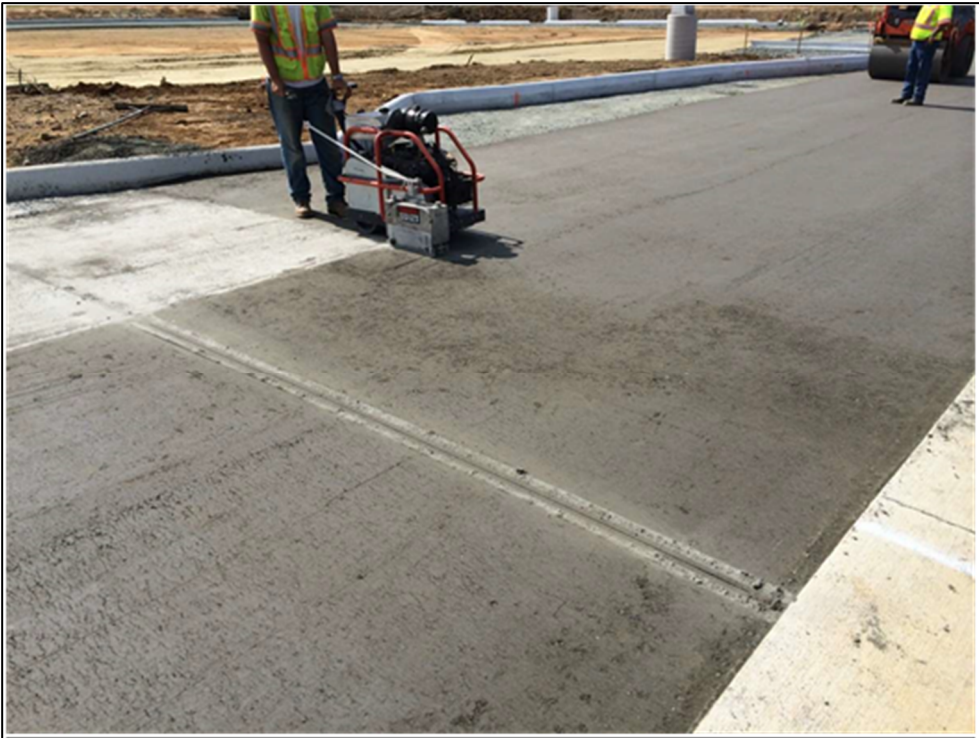
Joints are saw-cut.
