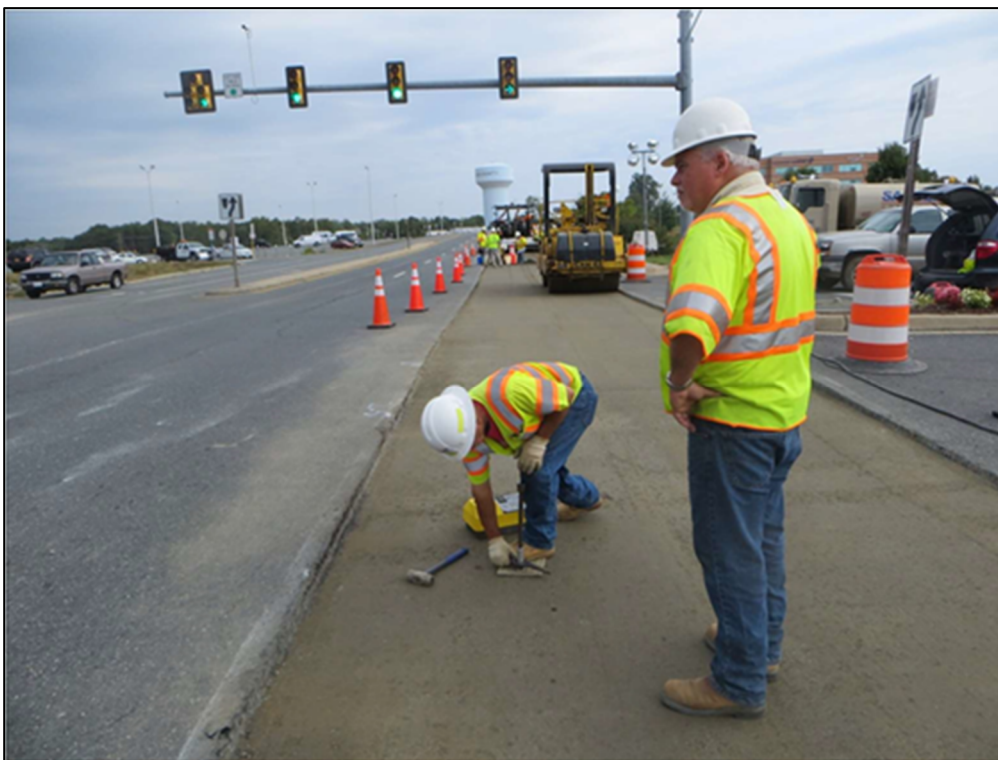
The density or compaction is checked with a nuclear density gauge.
