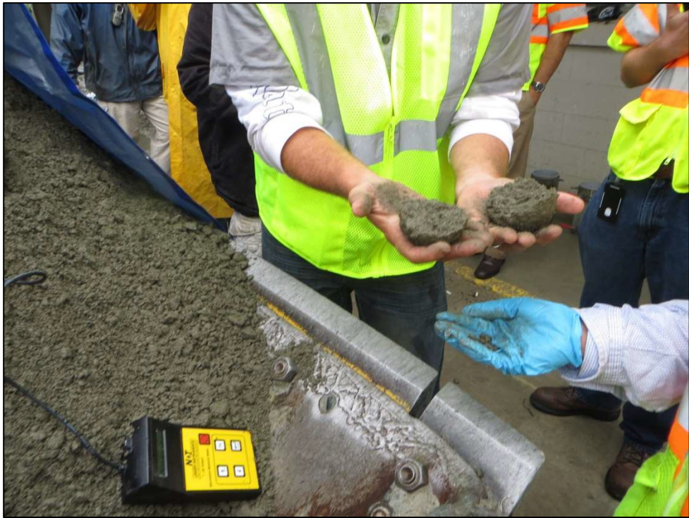
RCC looks dry.
