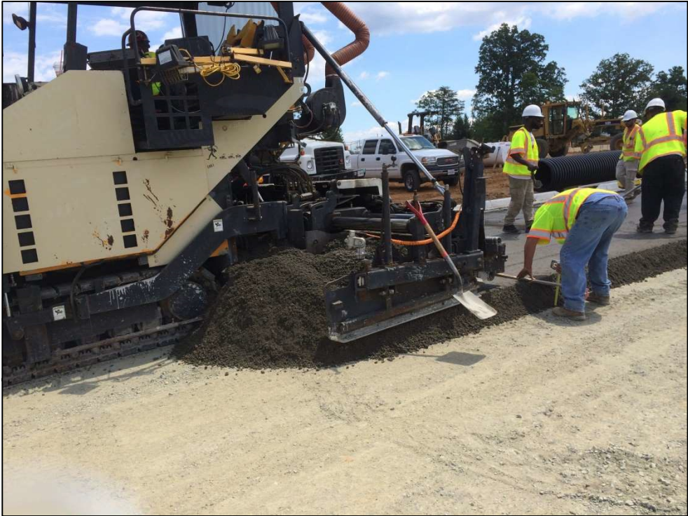
RCC placed with a high-density paver.
