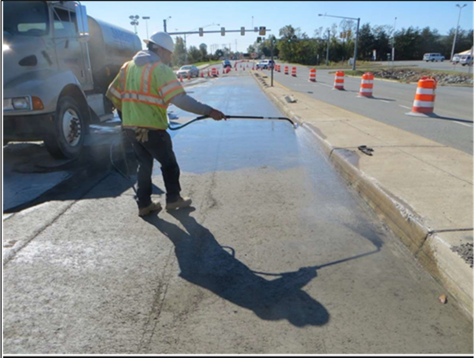
The concrete is kept moist during curing.
