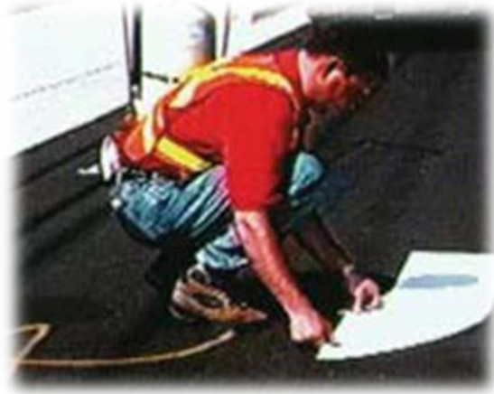
Figure 5.2 Placement of material
