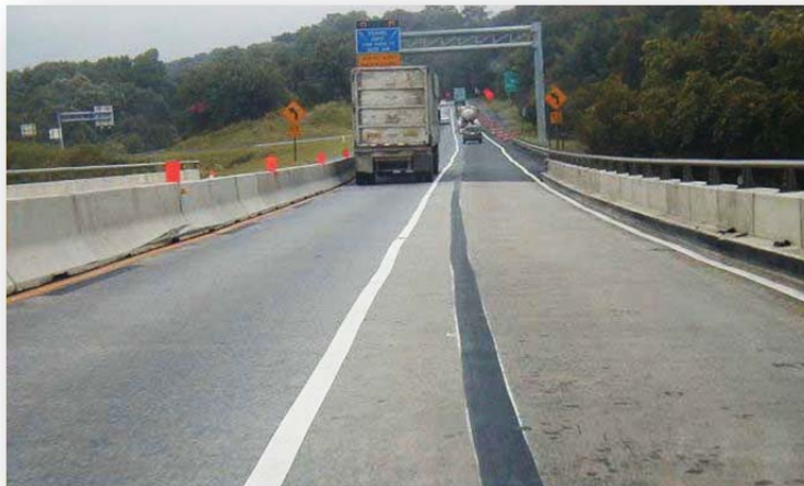
Figure 12.3 Black paint wearing off of previous marking
