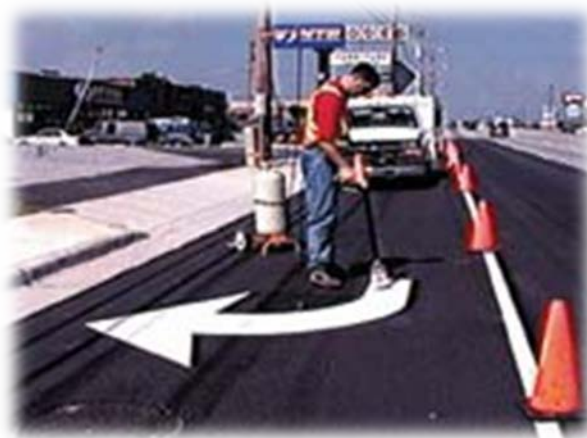
Figure 5.3 Arrow symbol being applied by heat torch.
