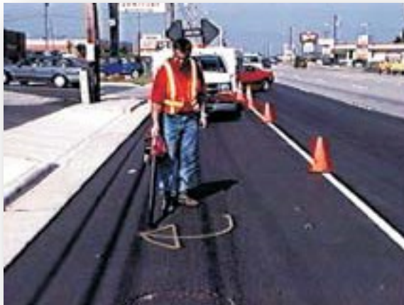
Figure 5.1 Cleaning pavement prior to application
