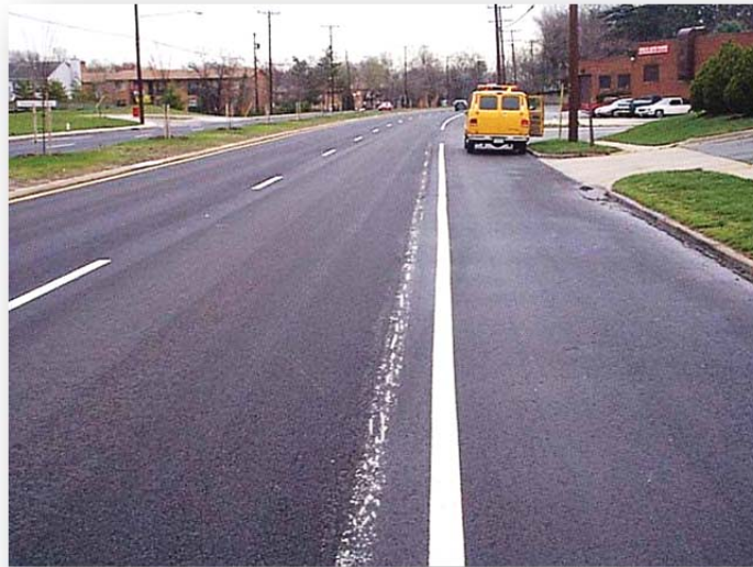
Figure 12.2 Scars from removed marking
