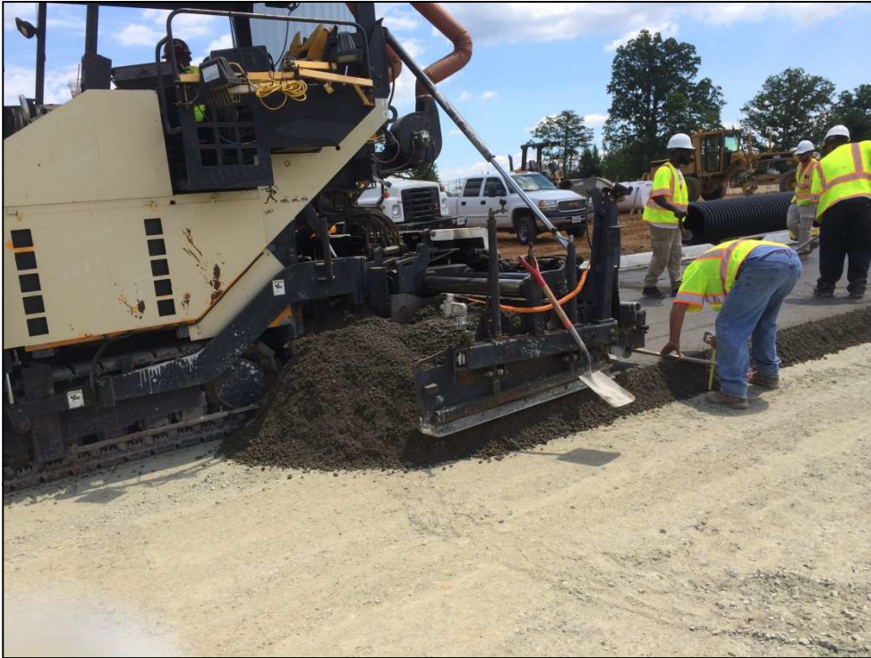
RCC placed with a high-density paver.
