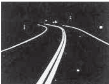
Figure 2.1 Pavement markings with reflective beads at night
