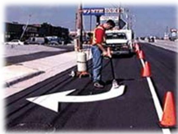
Figure 5.3 Arrow symbol being applied by heat torch.
