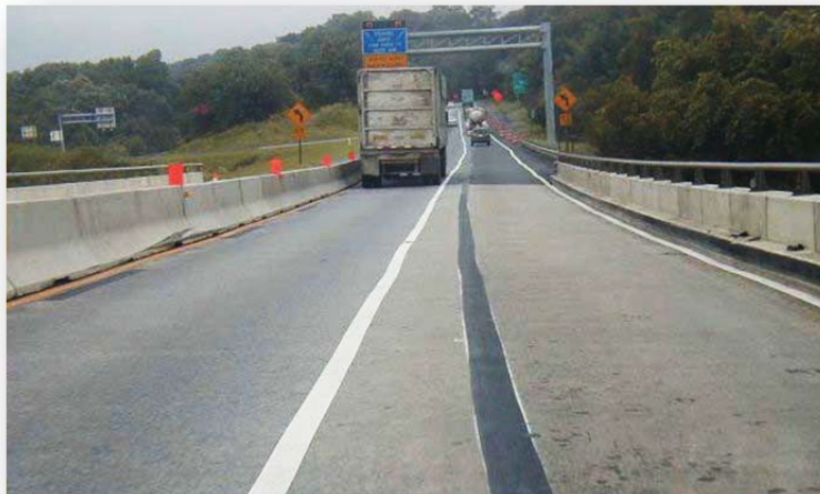
Figure 12.3 Black paint wearing off of previous marking
