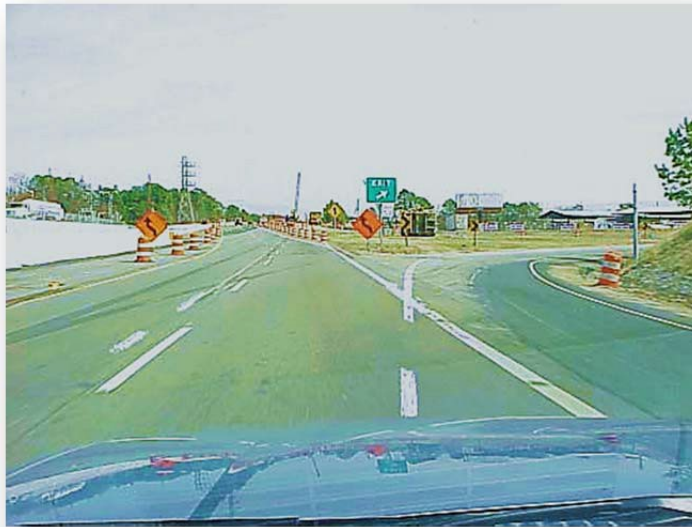
Figure 12.1 Roadway with confusing multiple lines
