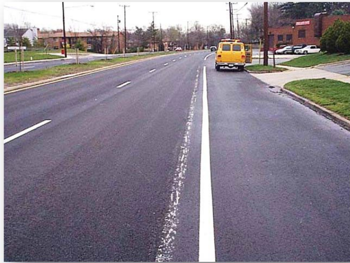
Figure 12.2 Scars from removed marking
