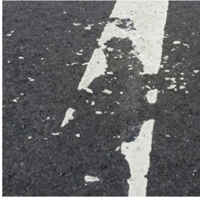
Results of shattering and poor bonding to the road surface.
